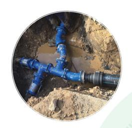
Working for Icon Water, ITS PipeTech were engaged to renew a 6.7 klm section of existing (CICL) Cast Iron main pipe in Canberra road, ACT. The system upgrade utilized **pipe bursting** technology to install a new replacement poly-ethaline pipe (PE) for the total distance of 6700 m through the City to minimize the disruption and interference to traffic and third party movement around the City
