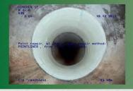
Point Lining is a localised structural repair solution which is installed over an identified defect, ensuring the pipeline is restored to its original operating condition. This widely used solution is approved for use in water catchment areas and is fully structural.
