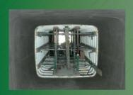
Tunneline is an exciting and innovative (patent protected) structural concrete lining system for renovating deteriorating and aging man entry pipelines, culverts and tunnels for water/wastewater, road and rail applications. Developed and widely used throughout the UK and Australia, the Tunneline process provides 100 year design life solution. Tunneline is designed to act as a standalone or composite liner in accordance with relevant Australian Standards (AS5100 and AS2566).
